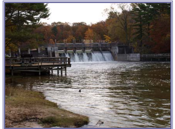
Hamlin Lake Dam photo by Bob Garrett
